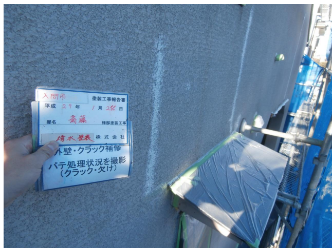
ひび割れ補修
